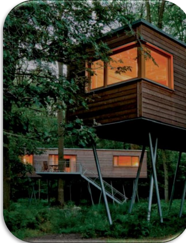
Outdoor construction in the middle of the forest, Resort Baumgefluester located in Bad Zwischenah, Germany close to the border with the Netherlands.
